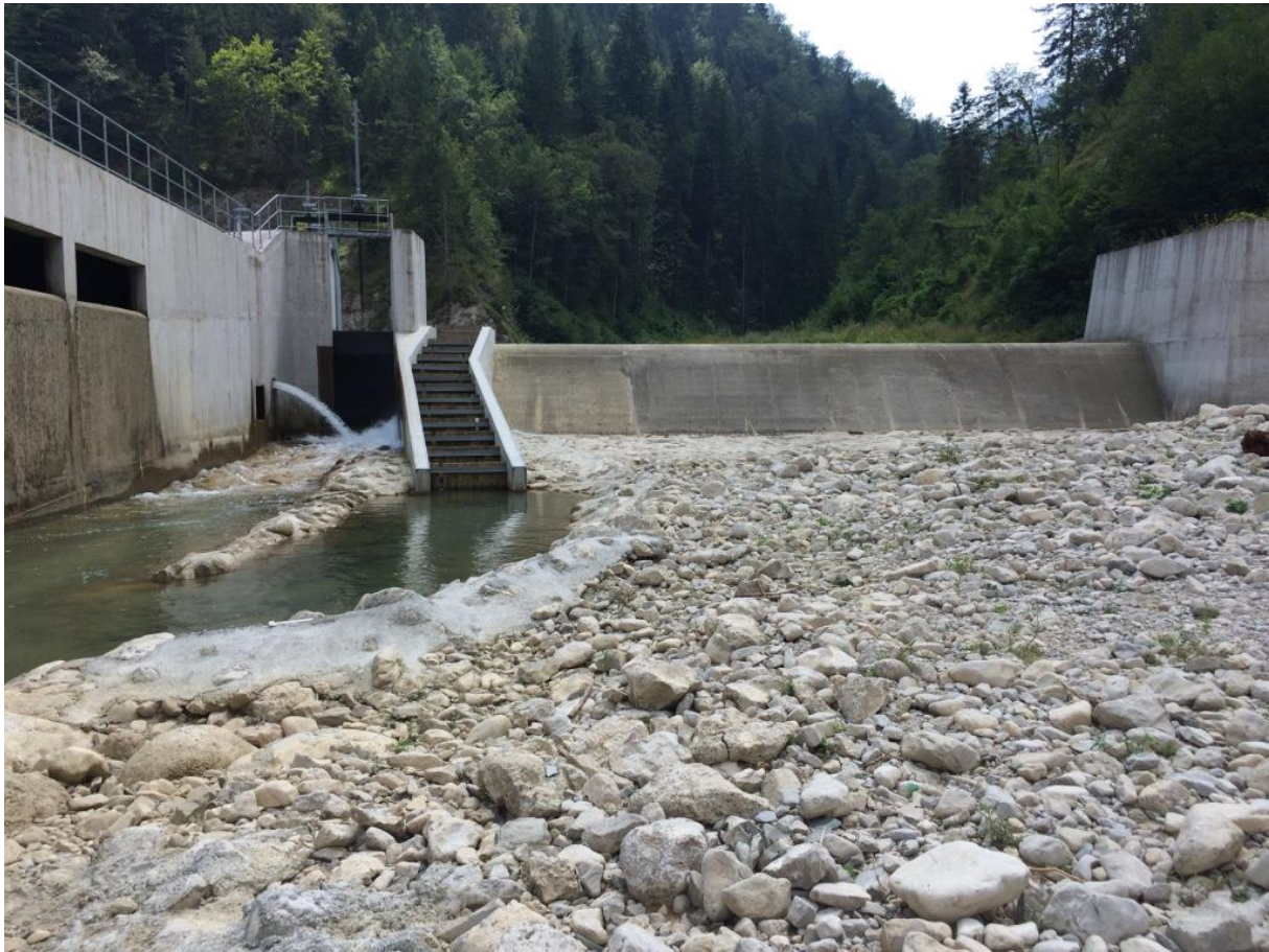
□ Figure 47: HPP Novakovici built by KELAG at the Ugar river in BA, a former huchen river. The fish ladder is inadequate and the residual flow downstream of the dam is insufficient - a trickle in the riverbed. (© Ulrich Eichelmann)
