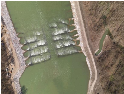
Figure 95: example of fish passable ramp of the river Salzach (Source Theo Steidl)
