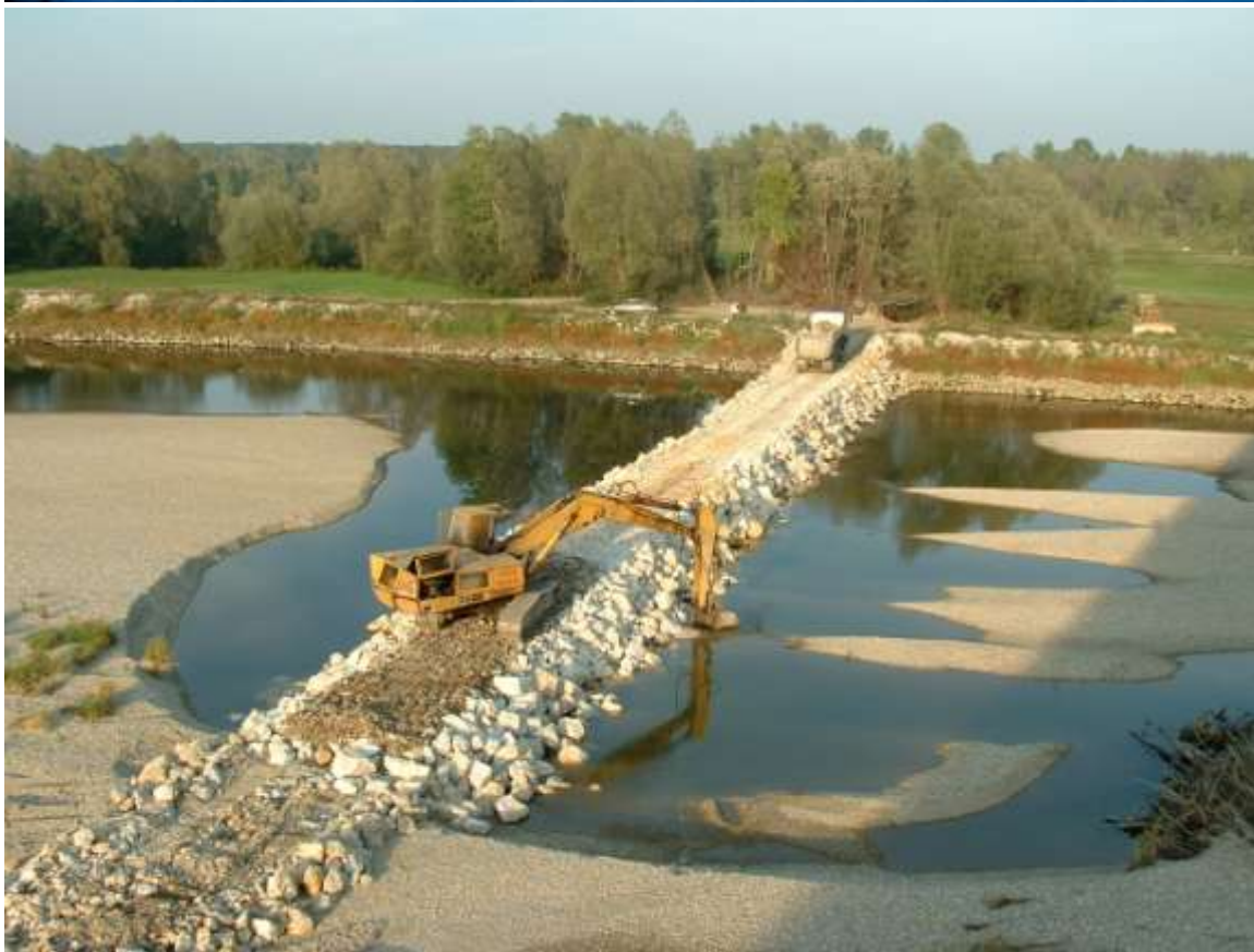
River regulation on the Drava, Croatia (Credit: A. Mohl/WWF)
