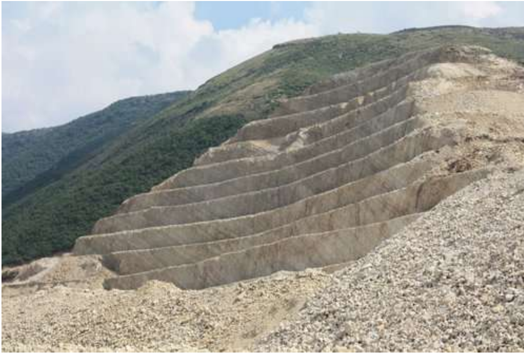
Vijosa (AL) dam under construction (Arno Mohl, WWF Austria)
