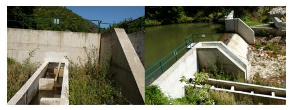
Figure 29: Blocked fish pass
