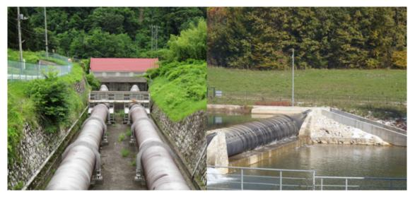
Figure 4: Pipes entering the powerhouse of a Figure 5: Ilovac run-of-the-river plant, source: TSREDCO Ltd. derivation plant. Author: Qurren
